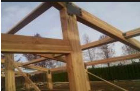
Mezzanine and shed rafter connection
