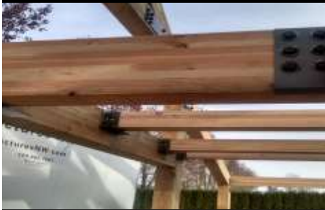
Mezzanine joist connection
